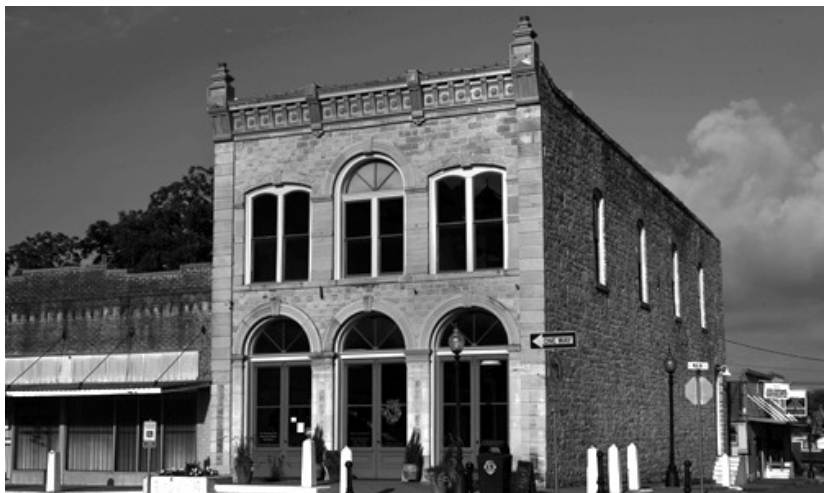
Gordon's 1890 Kahn & Stanzel Building, Hallettsville, Texas, Photo by Mieke Mahi
